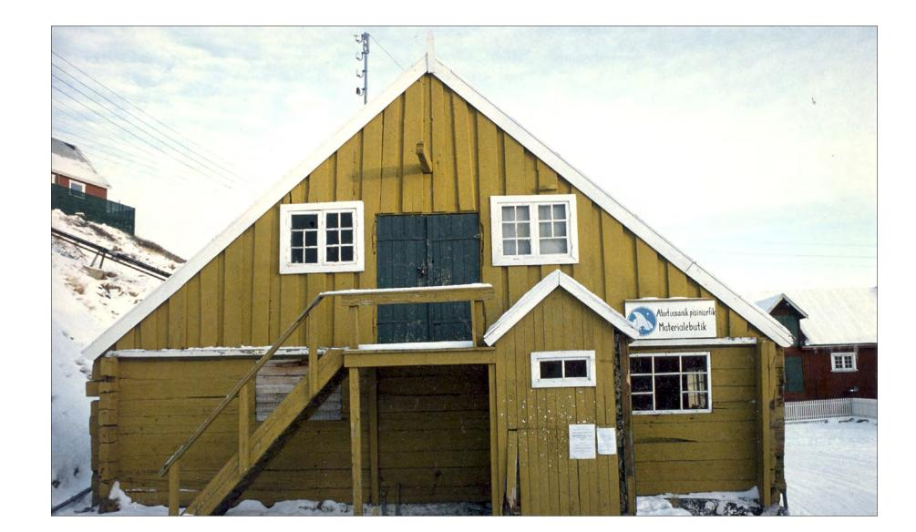
Helge Paulsen taking cores from house B-7 in Ilulissat, formerly owned by the Royal Greenland Trade *Company. 'Unscandinavian' construction details:* Logs are in line where they meet in the corners, and groove for timber list. Photo: Thomas Bartholin.
