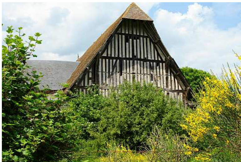
Aclou, Département Eure, Haute-Normandie. One of the few granges with external framework. Built in 1492(d)
